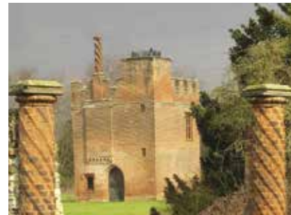
Gatehouse to Rye House, Stanstead Abbots, the home of Joyce Frankland
